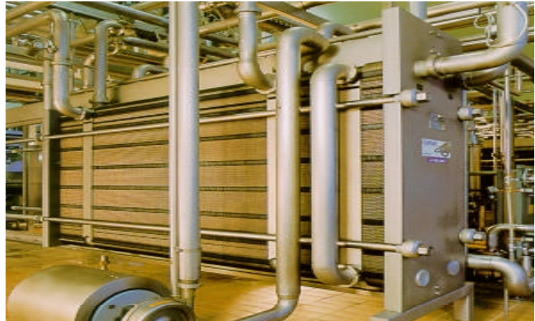
Figure 6.1 Plate heat exchanger .
