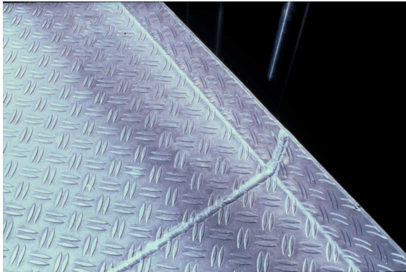
Figure 4.10 Materials used for staircases used must be easily cleanable but not slippery. Edge prevents transfer of soil towards product.
