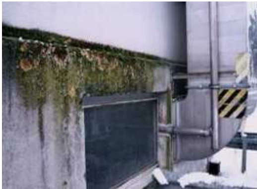
Figure 4.22 Left: bad location of intake opening of ventilation system. Right: air inlet not kept clean.
