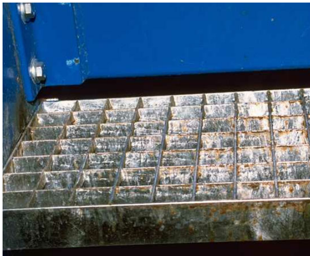
Figure 4.8 Open staircase (detail) with corrosion formation
