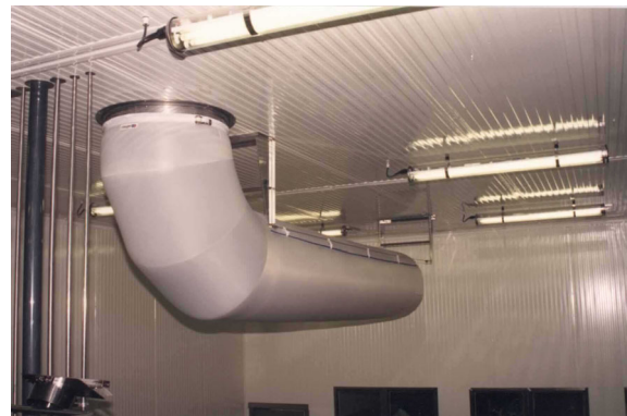
Figure 4.23 Air travels through a flexible airsock that can be removed and cleaned easily.
