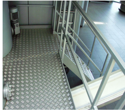
Figure 4.10 Materials used for staircases used must be easily cleanable but not slippery. Edge prevents transfer of soil towards product.
