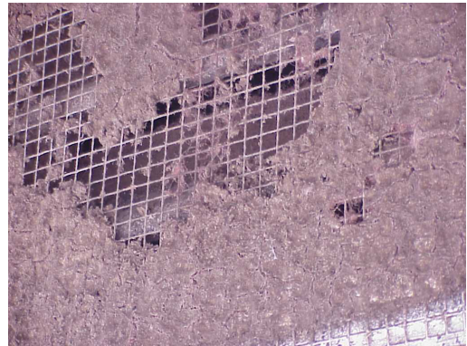
Figure 4.22 Left: bad location of intake opening of ventilation system. Right: air inlet not kept clean.
