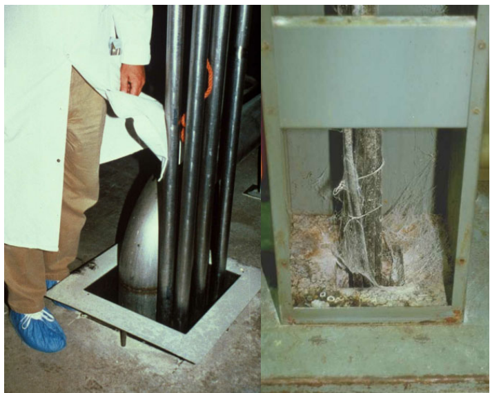
Figure 4.19 Openings for cables and pipes may be a source of contaminants and pests.
